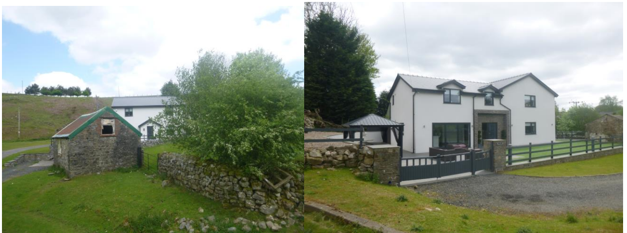
Figure 2. The existing outbuilding and the dwelling as constructed.
